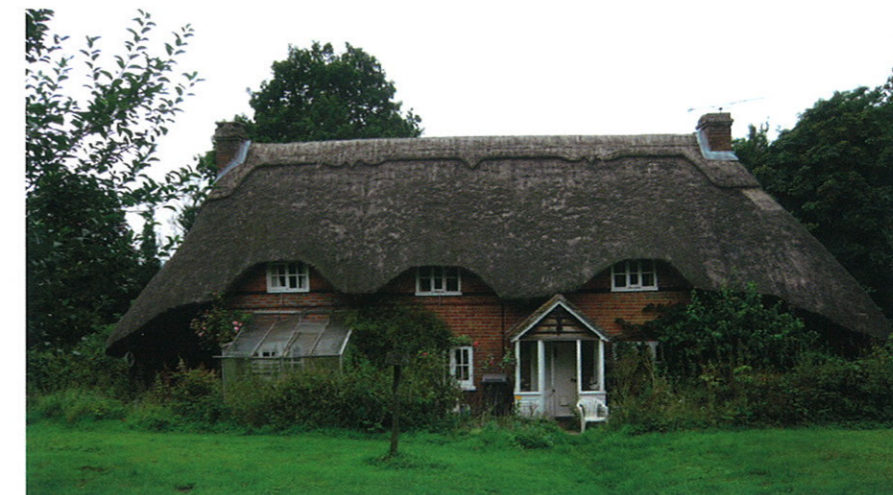
Fifteenth century unlisted cottage with long straw thatch, containing possible medieval basecoats, showing vermin runs below netted covering
