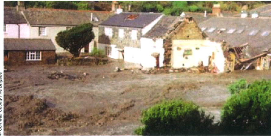
The destructive force of flood waters at Boscastle in 2004
