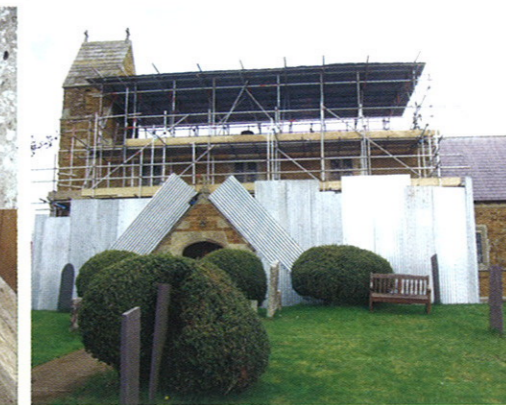
Enabling works associated with reroofing Photo by Barry Collins
