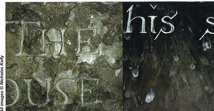
Image 1 – Difficulties in damage apportionment. Similarly dated wall plaques within the same major bat roost exhibiting dramatically differing damage: (left) the lower plaque within reach for cleaning is delaminating, (right) the upper plaque merely shows spotting
